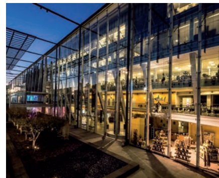
Building management platform Desigo CC at Museums Victoria
